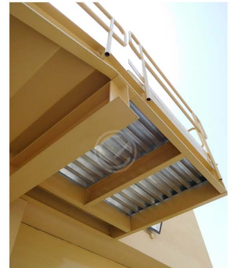
Concrete Stairs on Metal Decking
